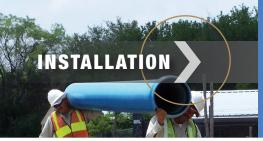
Lightweight, great for manual installation; no pipe puller needed.
