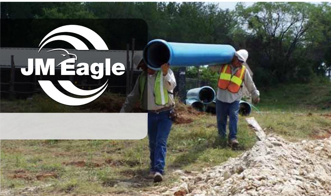
Since the PVCO pipe is specially manufactured to have a thinner wall, all while boosting strength, it is lighter than other comparable materials. Workers save time because they can move the 6-, 8- and 12-inch pipe without the help of heavy equipment.
