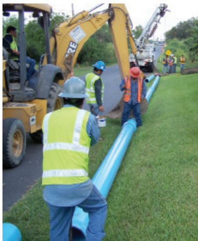
Figure 7: Example of an Eagle Loc joint assembly
